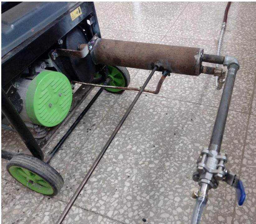
Figure 20: Corrected Alignment of bars on Manifold, Flue gas meter in the manifold (Source: Own Work)
