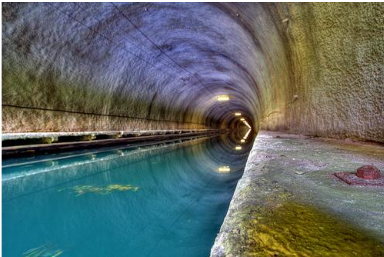
Figure 40 - Tunnel de Riqueval
